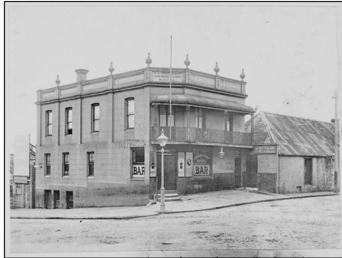
Figure 53 Balmain Ferry Hotel, Erskine Street c1907 (City of Sydney Archives)
