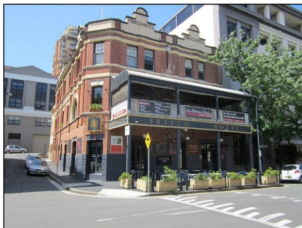
Figure 49 Frisco Hotel Woolloomooloo (History Services NSW)
