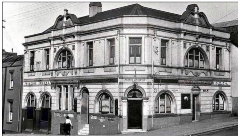
Figure 32 British Seamen's Hotel, Argyle Street (City of Sydney Archives)
