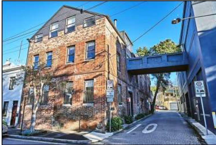
Figure 7 Former Acorn Pressed Metal Co (realestate.com.au)
