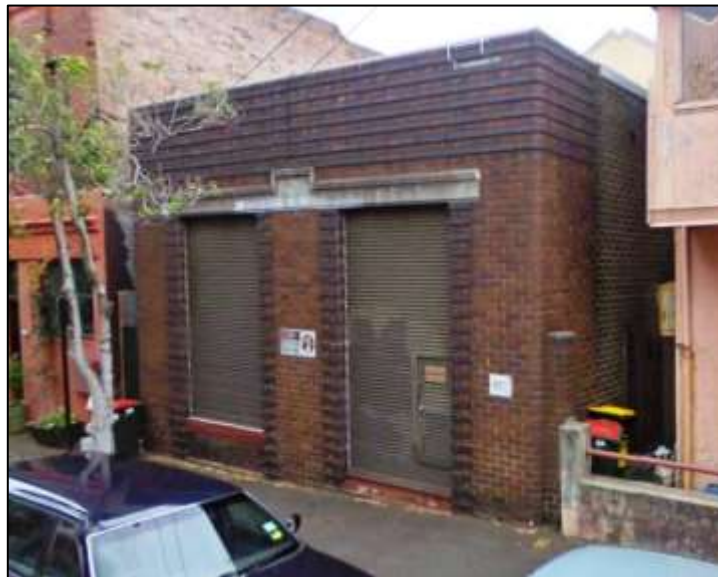
Figure 11 Electricity Substation No. 114 (Google maps)
