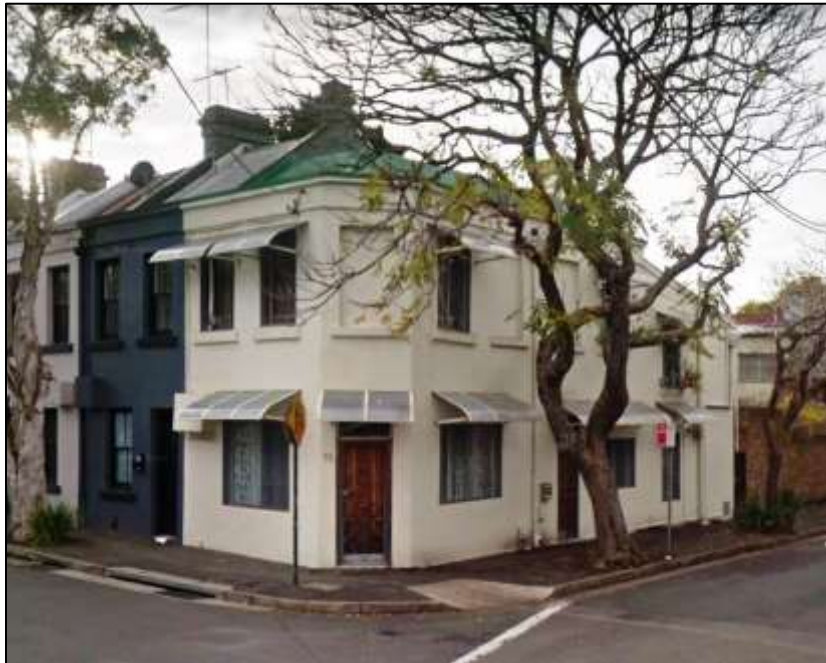
Figure 36 76 Marshall Street, 2015 (Google maps)
