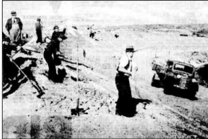
Figure 9 Demolishing the speedway, 1939 ( Sydney Morning Herald , 22 August 1939)
