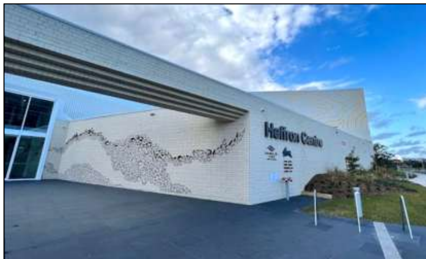
Figure 22 Heffron Centre (Randwick City Council)
