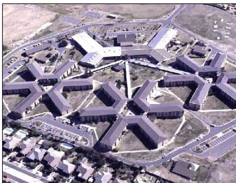
Figure 19 Endeavour Migrant Hostel, c1970 (National Library of Australia)
