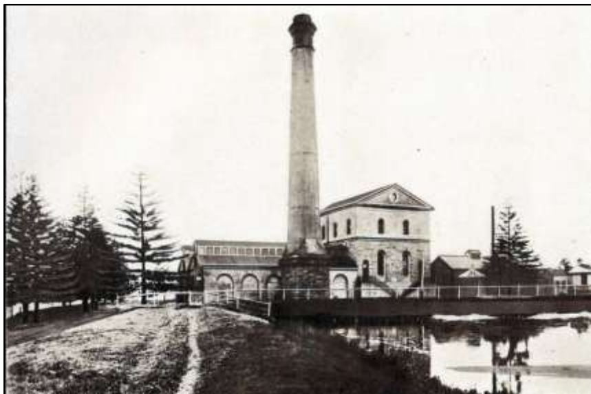
Figure 2 Botany Engine House (Sydney Water)
