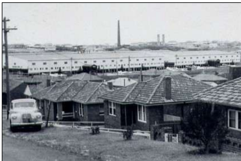
Figure 16 Matraville Migrant Hostel (Photo: Jo Mulholland)
