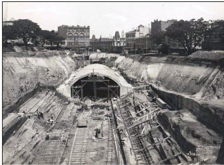
Figure 6 Tunnelling under Hyde Park, 1923 (Powerhouse Museum)
