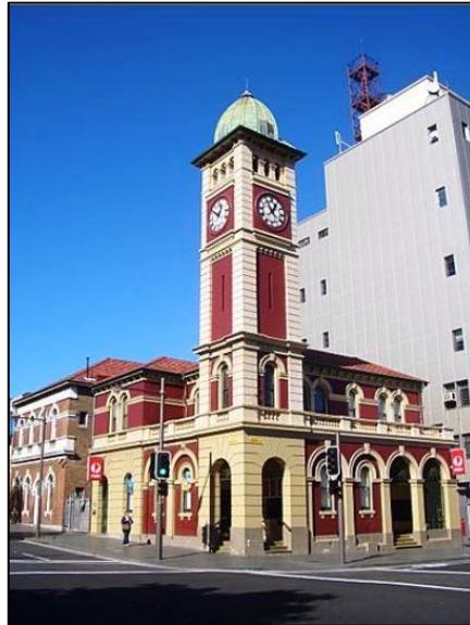
Figure 17 Redfern Post Office (Kiddle.co website)
